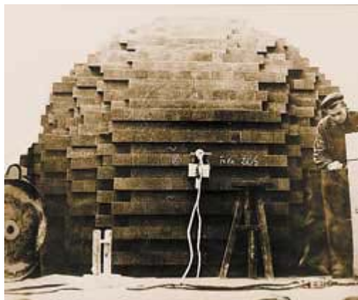
Figure 3.3. F-1: a dome of uranium bricks whose interior contained a neutron source. Sensors recorded the flow which reached to the surface. Photo from Larin I, 2010)
