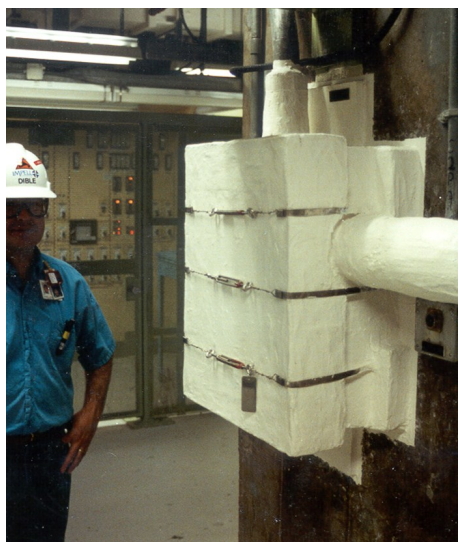
Fire-protected circuit. Photo courtesy NRC.
